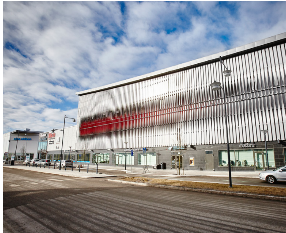
Paroc Built-on solution used in Ica Barkarbystaden, Sweden.
