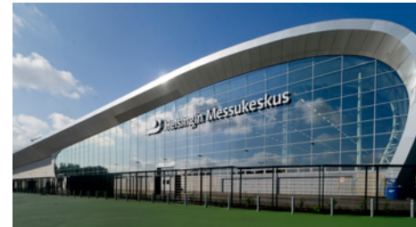
PAROC Cortex used in Helsinki Exhibition Centre Hall 7 walls.
