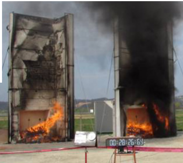
Fire Safe Europe organised a fire test in partnership with the Faculty of Civil Engineering of the University of Zagreb.
